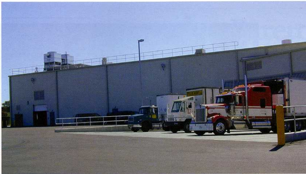
Freight haulers line up outside new, larger loading dock at Salida cold storage unit.
